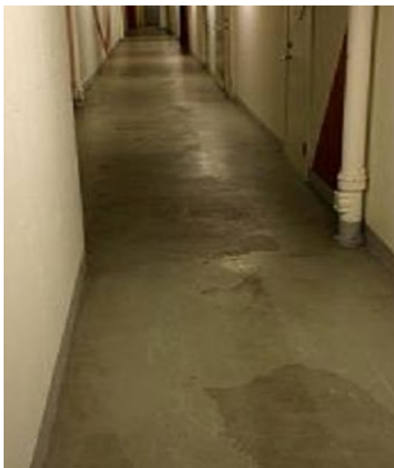
Before – Previous Painted with Epoxy Paint
